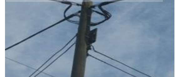
LOW VOLTAGE Concentric Neutral service cable
